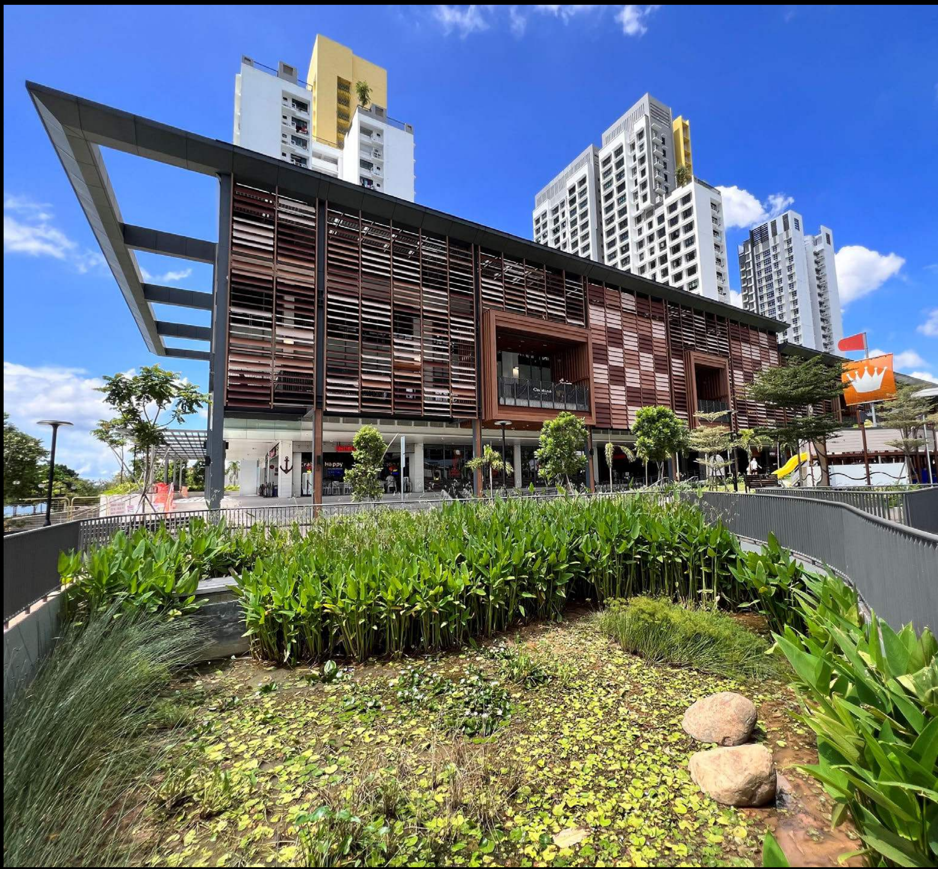
Northshore Plaza I & II – A naturally ventilated Neighbourhood Centre which was awarded with a Platinum Green Mark for its sustainable design
