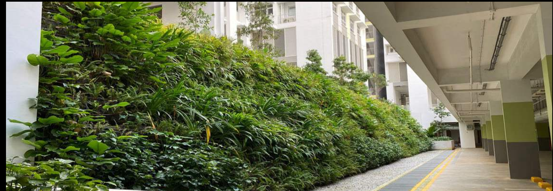
Geotextile bags are stacked and anchored at a slope of 70 degrees to replace conventional solution of a reinforced concrete retaining wall
